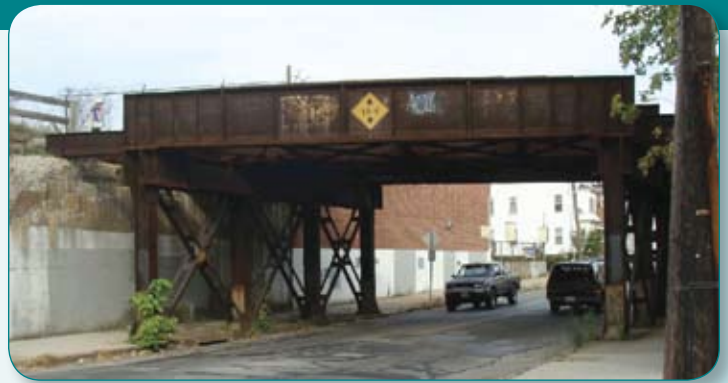
Sawyer Street bridge before reconstruction.
